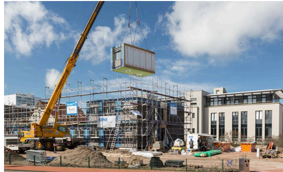
Piece by piece, the rehab centre was skilfully assembled from individual modules (© ERNE AG Holzbau | photograph: Jan Meier, Bremen)
