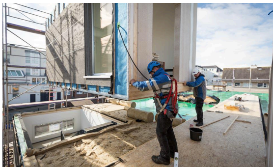
Piece by piece, the rehab centre was skilfully assembled from individual modules (© ERNE AG Holzbau | photograph: Jan Meier, Bremen)
