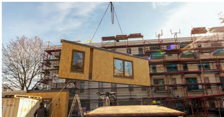
Placing the prefabricated walls made of SWISS KRONO OSB
