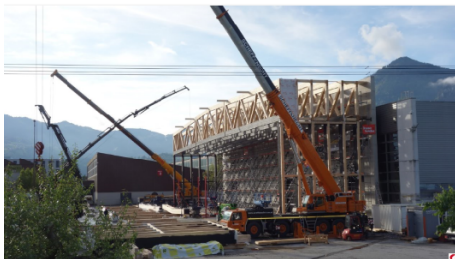
Both the loadbearing walls and the ceiling construction are being made using timber and engineered wood products (photograph courtesy of: Messe Dornbirn GmbH)
