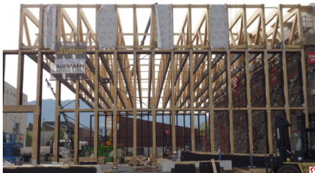
Both the loadbearing walls and the ceiling construction are being made using timber and engineered wood products (photograph courtesy of: Messe Dornbirn GmbH)
