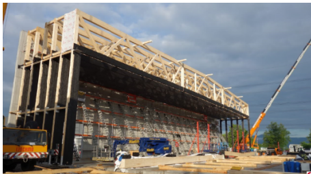
The halls going up: 66m-long beams without any supports in the middle (photograph courtesy of: Messe Dornbirn GmbH)
