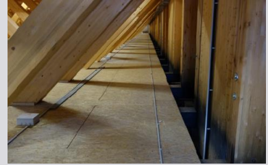
OSB boarding resting on the bottom chords of the roof truss
