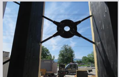
Connecting eye of steel braces for reinforcing a wall
