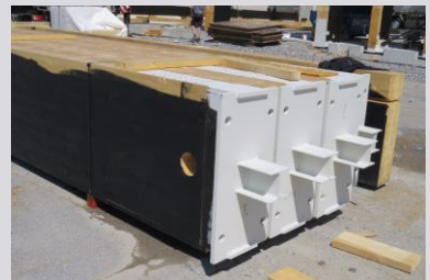
Details of the loadbearing glulam posts for the exterior walls
