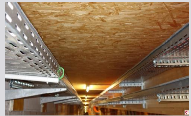
Installation shafts beneath the roof members
