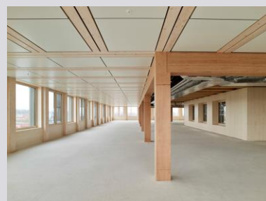
Visible birch wood columns and struts provide an enhanced aesthetic effect. (© ERNE AG Holzbau | Photograph: Markus Bertschi)
