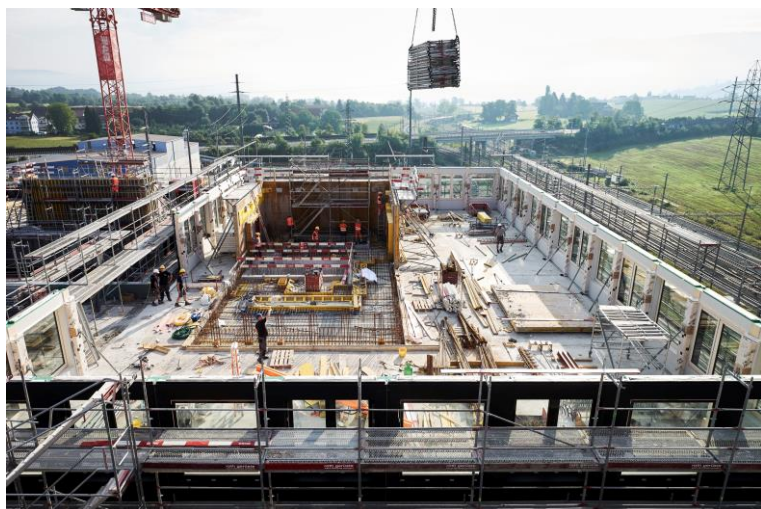
Start of construction of the 10-storey, 36m-high hybrid tower in August 2016. (© ERNE AG Holzbau | Photograph: Markus Bertschi)
